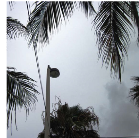
Fig. 4 - Type 3 Street Light located adjacent to the south of the FAU SeaTech campus.
