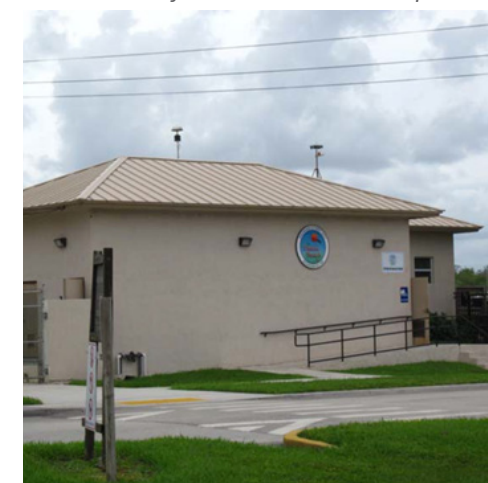
Fig. 6 - Exterior lighting at current dock master's office.
