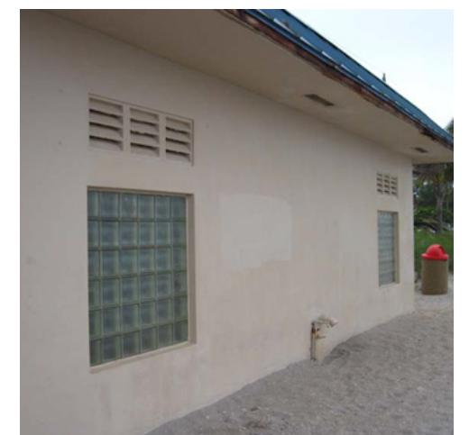
Fig. 7 - Beachside of existing northernmost restrooms.
