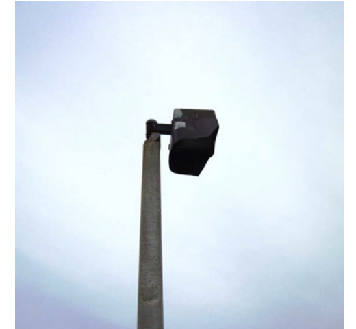
Fig. 3 - Type 2 Street Light located within the parking lot
